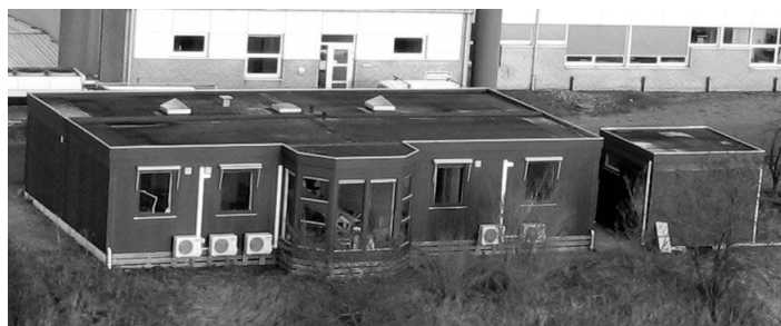
Figure 6. The PowerFlexHouse building.
