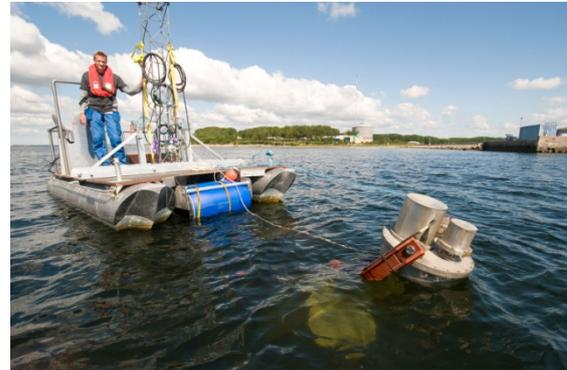
Figure 8 Demonstrator foundation with mast in position 50m from pier, torque arm is lifted with generator box above sea level and sea vessel surrounds mast
