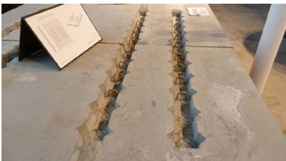
**Fig. 8** Grooves for slack reinforcement at top of a SL-deck for a joint with another element.
