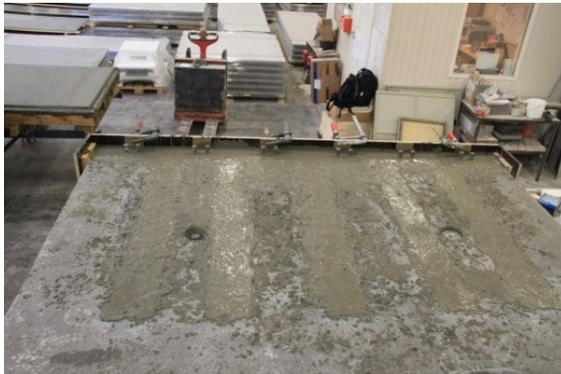
Fig. 16 Cast out joint and grooves.
