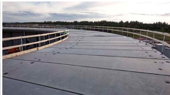
**Fig. 5** Wedge shaped SL-Deck elements with rounded ends making a circular building for Innovest 2014. Architect Aarstiderne.
