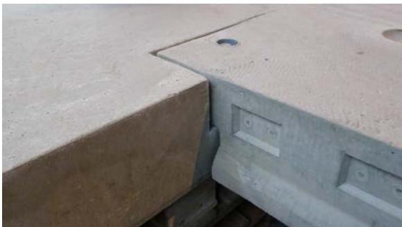
**Fig. 4** SL-Deck element with blade connection supporting it on the side of another SL-Deck element.
