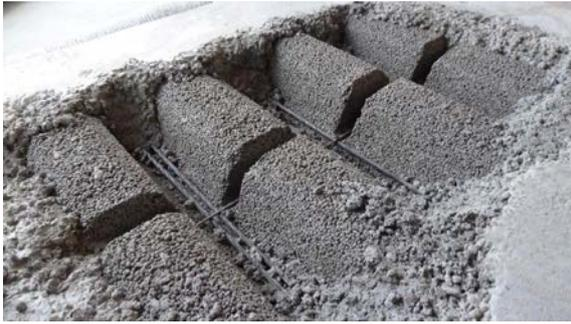
**Fig. 2** SL-Deck Element illustrating the construction by visible light weight aggregate concrete blocks, pretensioned tendons and cross reinforcement.
