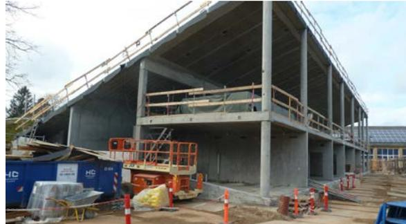
**Fig. 3** SL-Deck elements with blade connections and a sound damping part of bottom surface for the class rooms at Old Hellerup High School 2014. Architect BIG.
