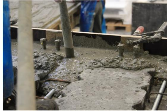
Fig. 15 Casting of joint and top grooves.
