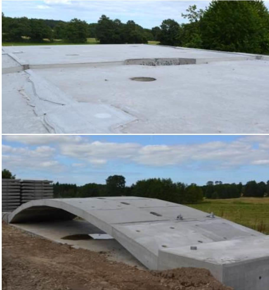
**Fig. 8** Top: Close up of difference in height between the two arches at the crown showing the requirement of high accuracy during the assembly process. The first arch (closest) was placed on the foundation three weeks prior to the second arch (furthest away). Bottom: The first 13 m span PC arches in their final position.
