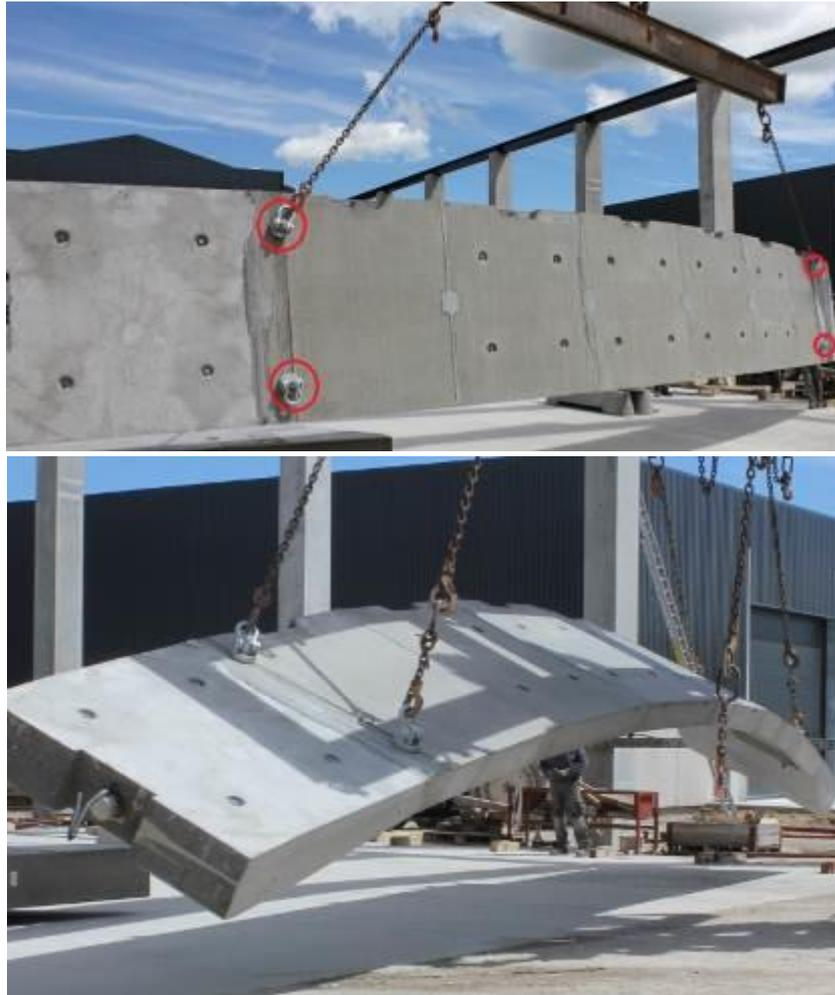
**Fig. 4** Top: Lifting points for PC arch (circled in red). The two top points were used for the initial vertical lift. Bottom: Subsequently, the two bottom lifting points were connected, and the arch was rotated, positioned on temporary supports, and transported by truck to the erection site.
