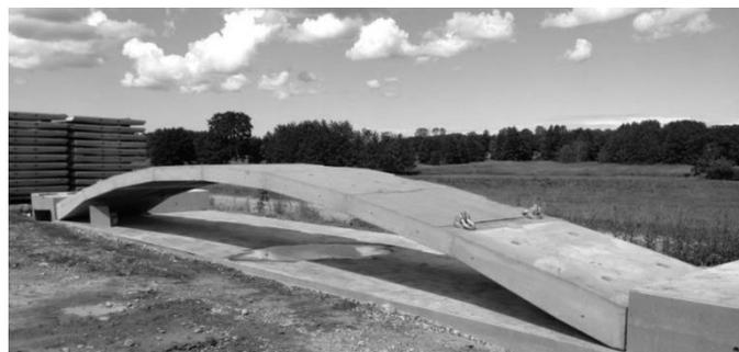
**Fig. 2** After casting the mortar joints and post-tensioning the Pearl-Chain Bridge arch substructure, it is placed in position by a crane. The photo shows a test arch with a span of 13 m and a width of 1.75 m. Several arches can be placed next to each other to provide the necessary width of the bridge.
