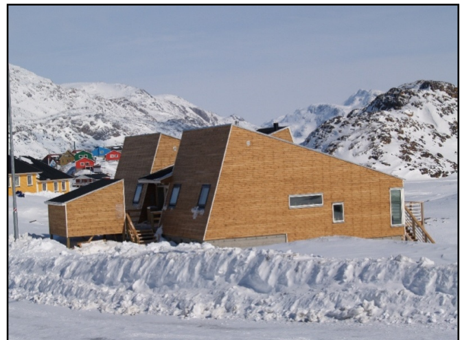
Fig. 1. Photo of the low energy house in Sisimiut as seen from the west.
