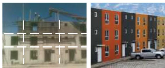
Figure 2: Standardized concrete segments applied at Victoria
