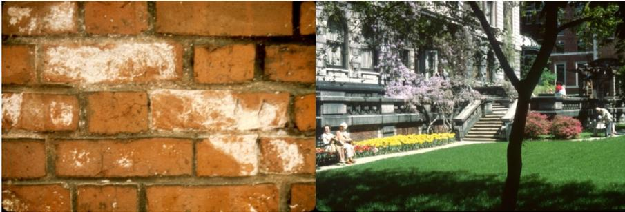
**Figure 2:** Detail of the brick wall showing the gypsum efflorescence formed on the parallel wall below grade to that seen in the garden at right.
