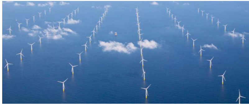
Figure 2. Gemini wind farm located to the North of the Netherlands; this wind farm contains 150 Siemens 4MW turbines. Courtesy: Van Oord.
