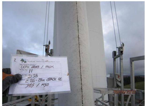
Figure 3 Front edge cracks (transverse and longitudinal)
