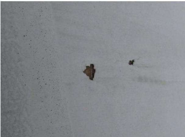
Figure 6 flaking of the top coat
