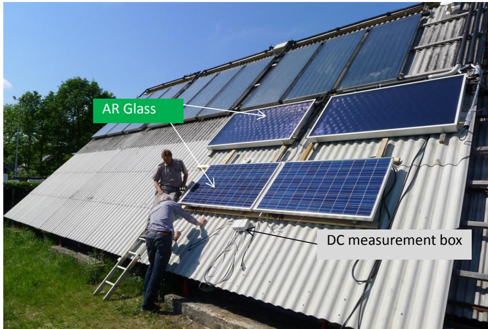
Fig.1. The PV modules during installation in May 2013. Above the PV modules, thermal collectors with the same glass types can be seen.
